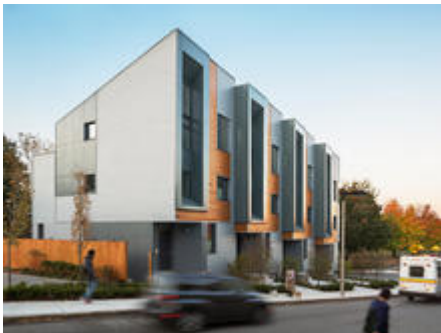
View West Along Highland Street - Photo Credit: Sam Oberter
