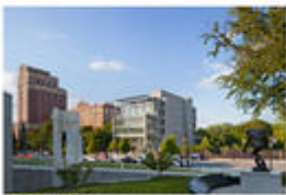
Exterior Elevation Photos - Photo Credit: Perkins+Will
