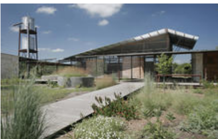
Covered Entry Plaza - Photo Credit: Stephen Miller
