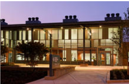
Solid portions of the curtainwall are filled with 6" of spray foam insulation for a 30% window to wall ratio. - Photo Credit: Stephen Miller
