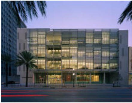
Exterior View from Canal Street - Photo Credit: Timothy Hursley
