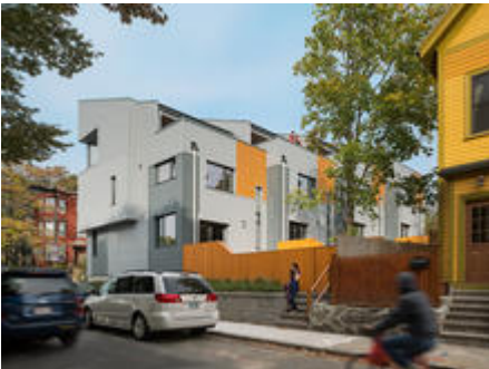
Rear Facade from Marcella Street - Photo Credit: Sam Oberter
