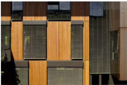
Dynamic exterior blinds keep unwanted sun out of southwest-facing interiors. - Photo Credit: Jeremy Bittermann
