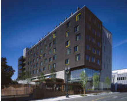
View of Bud Clark Commons from the northeast, including custom entrance gate that leads to public courtyard for the homeless seeking services and shelter. - Photo Credit: Sally Schoolmaster
