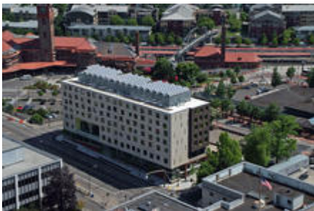
Aerial view of Bud Clark Commons' onsite PV array. - Photo Credit: SkyShots
