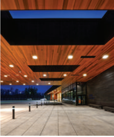
Secondary Canopy and Main Public Entrance - Photo Credit: Paul Crosby
