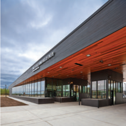
North Facade and Primary Inspections - Photo Credit: Paul Crosby
