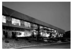
Light shelves (on the lower level) and shading devices help make this conventional tilt-up concrete building energy efficient. - Photo Credit: Miller/Hull
