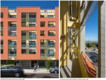
LEFT: Southwest facade with living screen wall; RIGHT: Southwest balconies behind a living screen wall - Photo Credit: Tim Griffith
