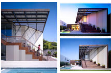
Views of SE portion of house - Photo Credit: John Linden
