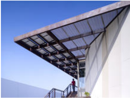
Detail of the large southwestern overhang with the 12kw solar system - Photo Credit: John Edward Linden
