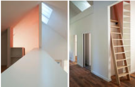
View from loft over top of marriage wall (left). Integrated ladder allows access to loft (right). - Photo Credit: Ken McCown
