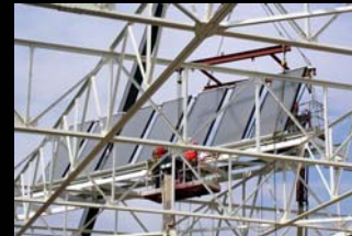
solar panel installation
